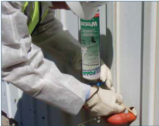
Filling & sealing small annular through-wall penetrations
