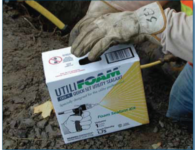
Plug open ends of abandoned mains, service piping and conduit
