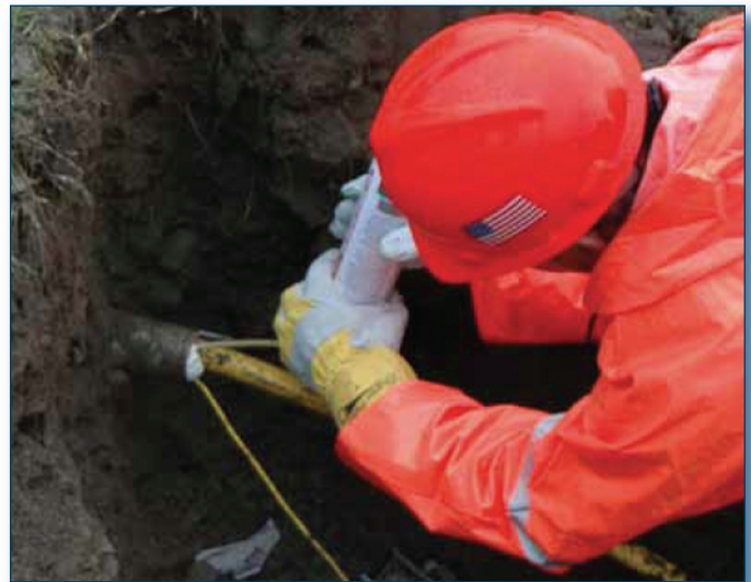
Filling & sealing service line insertions
