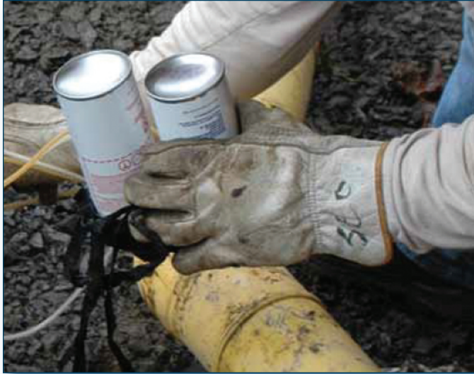
Plug open ends of abandoned mains, service piping and conduit
